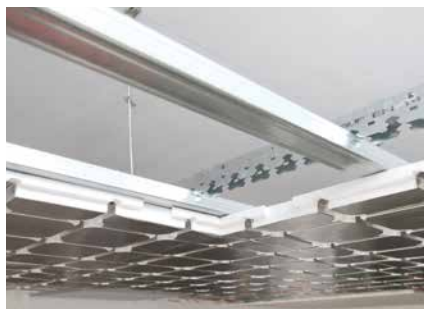
Installation of metal structure with 300 mm pitch
