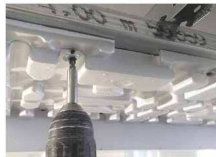
Installation and fitting of head panels on the metal support structure with 35 mm screws
